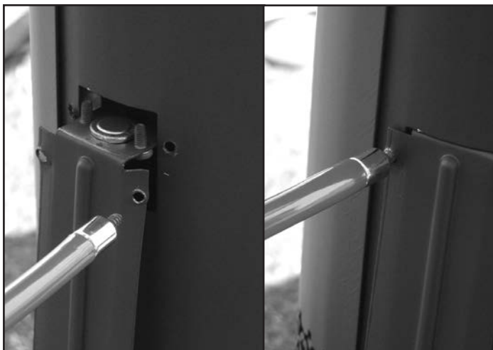
Figure 49: Spill switch installation.
