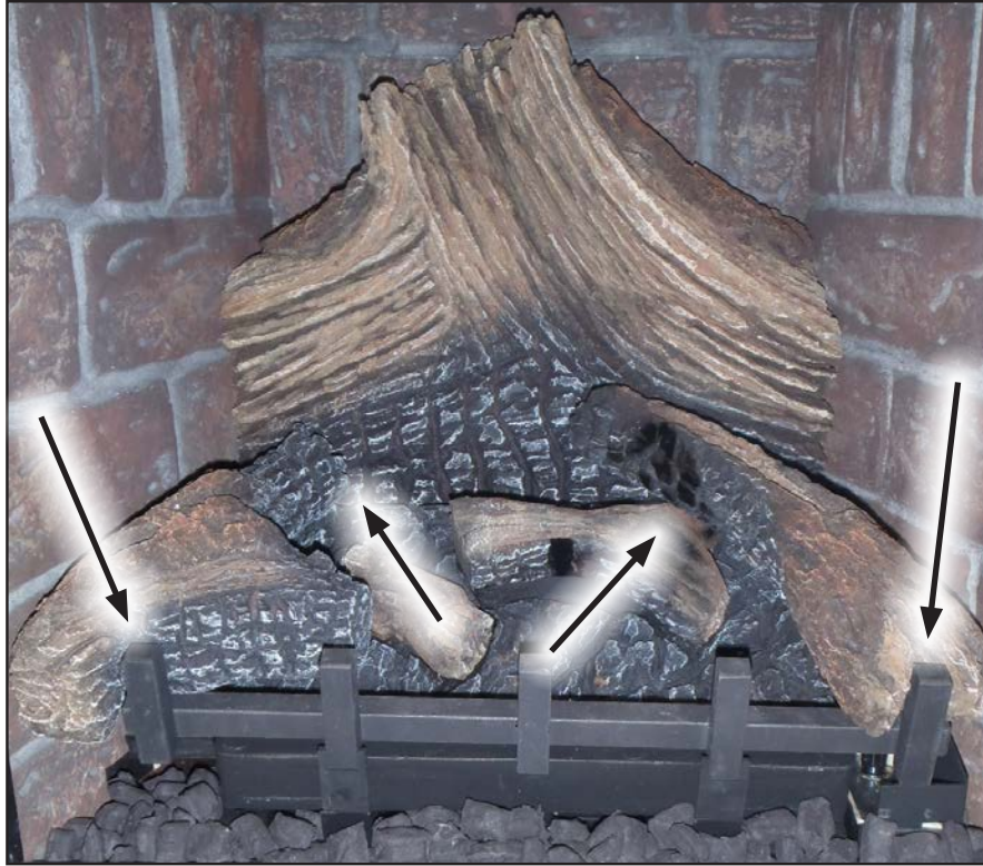
Figure 38. Third Stage Log Set Installation.
