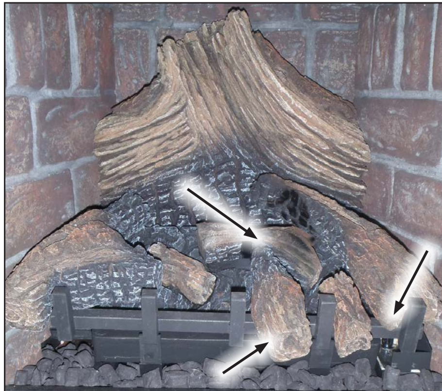
Figure 39. Fourth Stage Log Set Installation.
