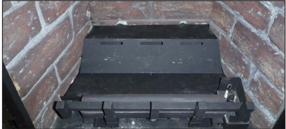
Figure 35. Empty firebox with grate and locator pins.
