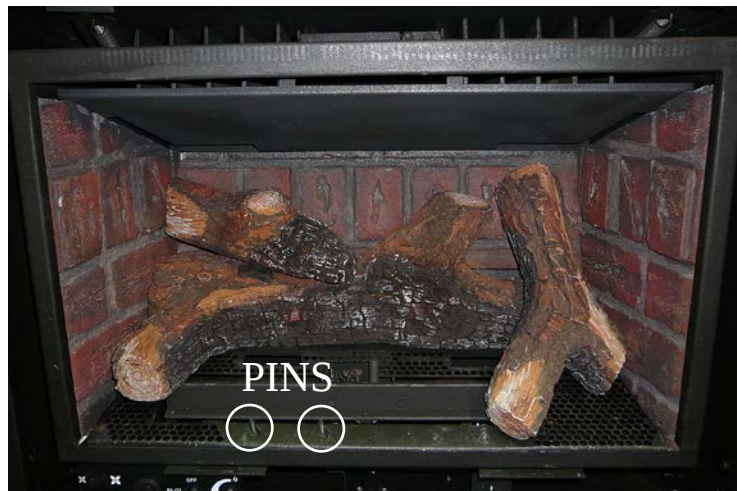
Figure 70. Third Stage Log Set Installation.
