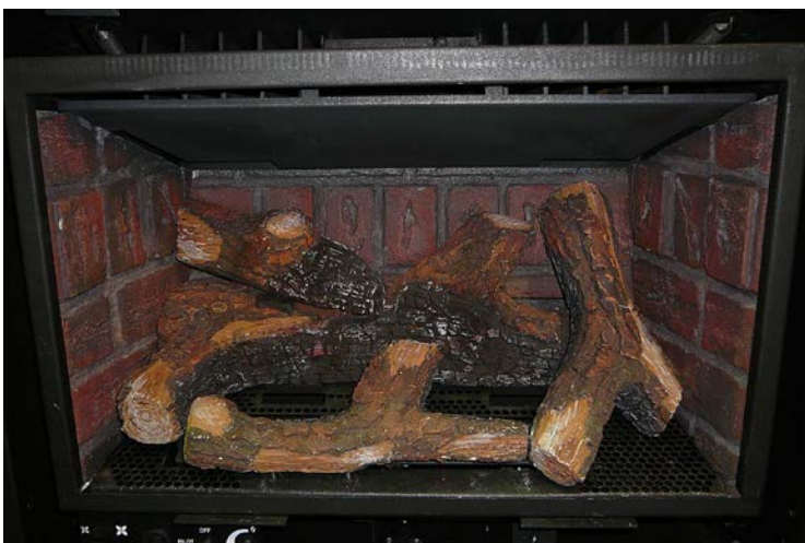
Figure 71. Fourth Stage Log Set Installation.
