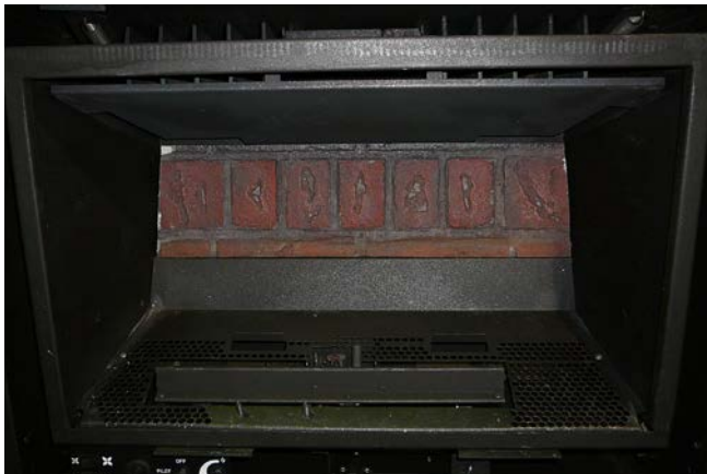
Figure 65: Back Brick Panel in Place.
