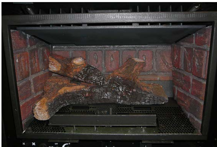
Figure 69. Second Stage Log Set Installation.
