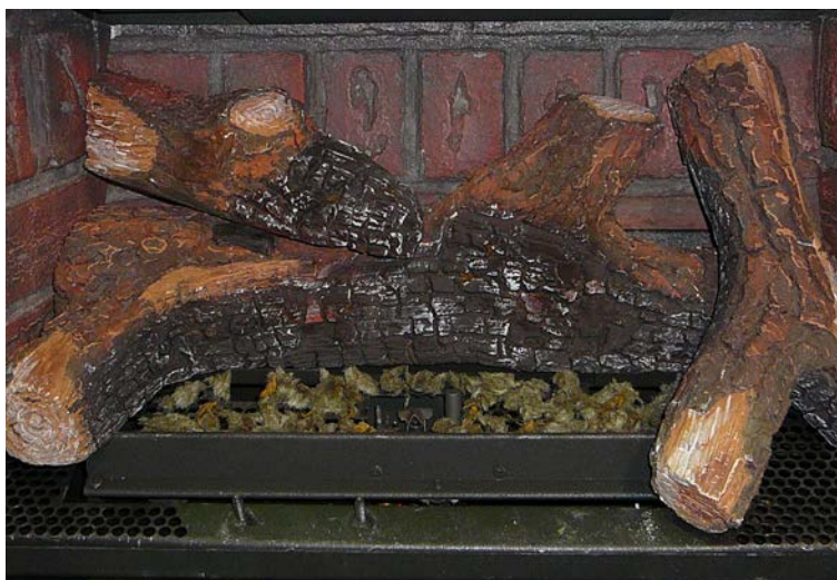
Figure 72. Fifth Stage Log Set Installation.
